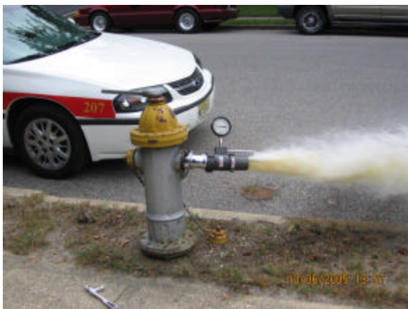
Figure 4: Hydrant flowing water. Gauge is reading residual pressure.
